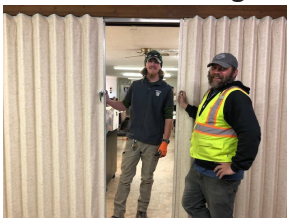
New folding Door installed
